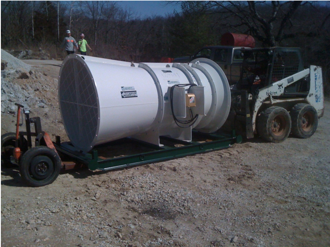
Figure 7.8. Booster fan transportation
